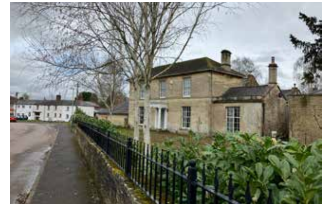
Figure 15: Low rise wall with black metal railing clearly delineating the edge of pavement.
