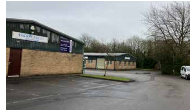
Figure 50: Neighbouring industrial units and the adjoining car park, east of the site
