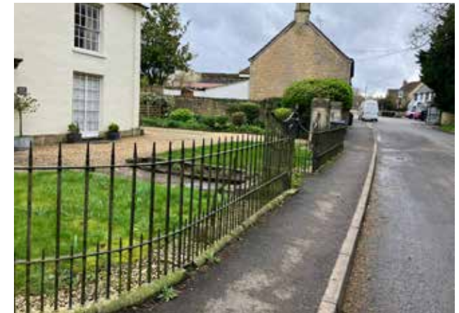
Figure 24: A clearly marked, but narrow pavement, High St
