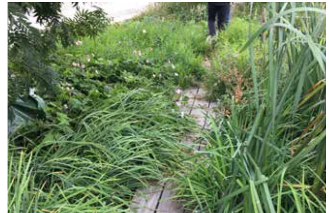
Figure 35: Example of SuDS designed as a public amenity and fully integrated into the design of the public realm, Stockholm.
