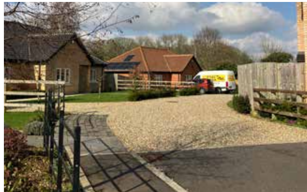
Figure 67: Application of permeable and contrasting surface in a shared street, Strumpshaw.
