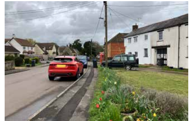
Figure 11: Consistent building heights along the High Street
